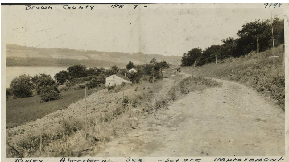
A photo from the Ohio Department of Transportation's archives. This photo from 1926 shows SR7 road in the Ripley Aberdeen area.
